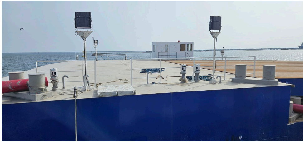
Fig. 1 Current pontoon structure in use for ro-ro ship mooring operations
