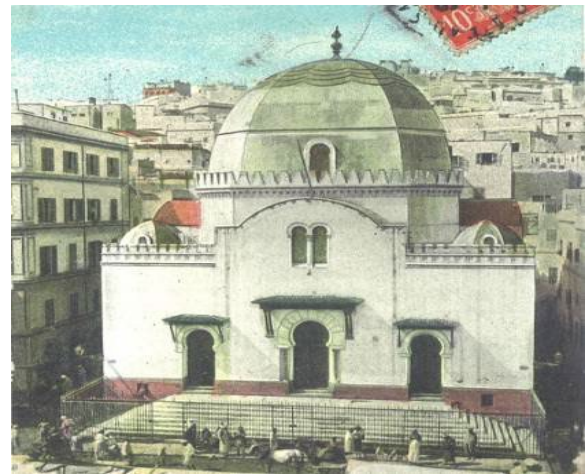
Figure 1: Main façade of the synagogue of Algiers
