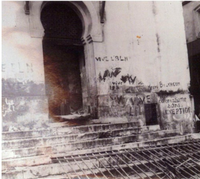
Figure 3: The deterioration of the Great Synagogue in 1961
