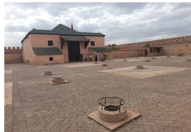
Entrance view of Quara Prison (Meknes)
