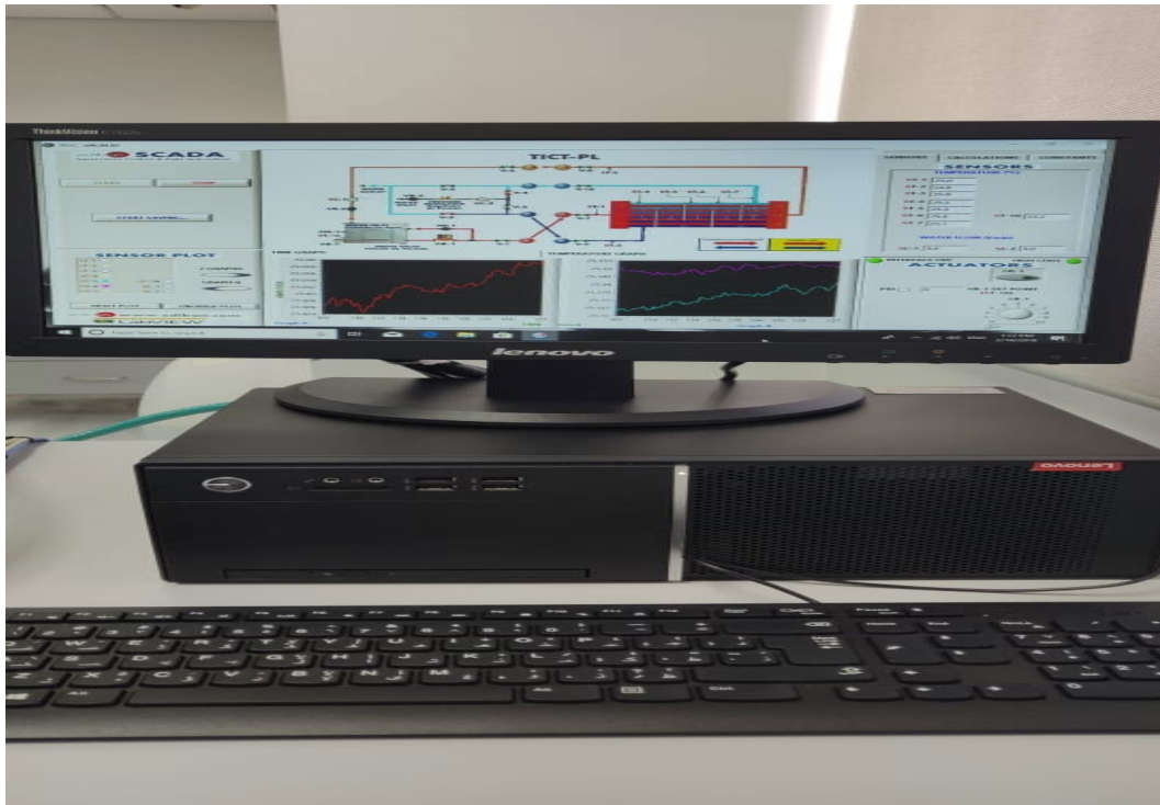
Figure 2. PLC-SCADA Data recording and process monitoring system
