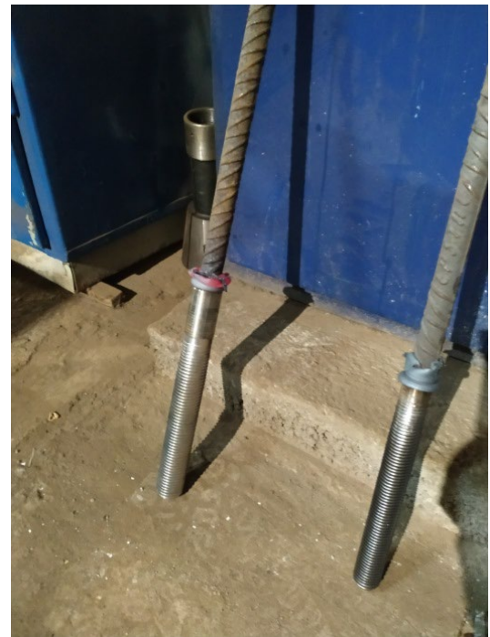
Fig. 1. The joint after welding
