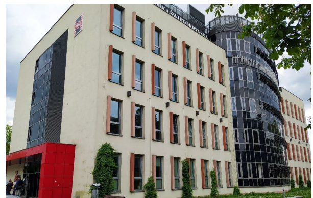
Fig. 2. Photo of the Energis building.
